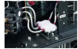
Coated Electrical Connections
